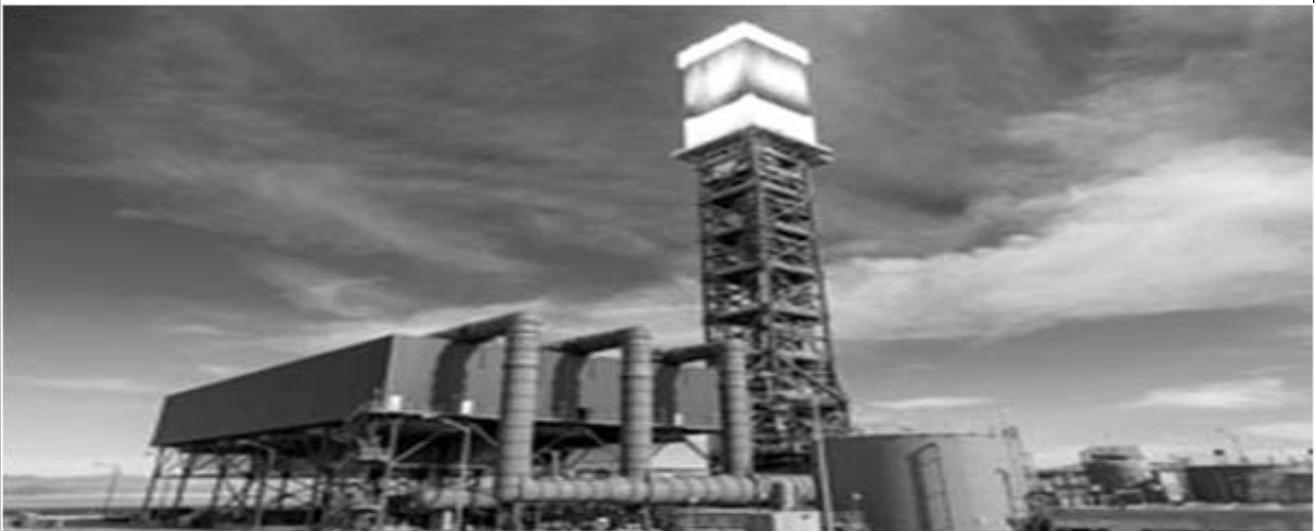
Ivanpah Solar Electric Generating System situated in the Mojave Desert in California is the World's largest solar power plant. An engineering marvel in itself, Ivanpah uses over 3,00,000 mirrors (heliostats) to reflect heat and light from the Sun onto boilers atop three of the towers here. Each of these towers is 150 feet taller than the Statue of Liberty.
