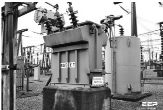
Earthing (grounding) transformer – Voltages during a ground fault.
