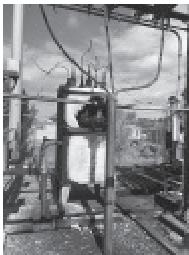
Figure 1 - Explosion of an oil in circuit breaker
