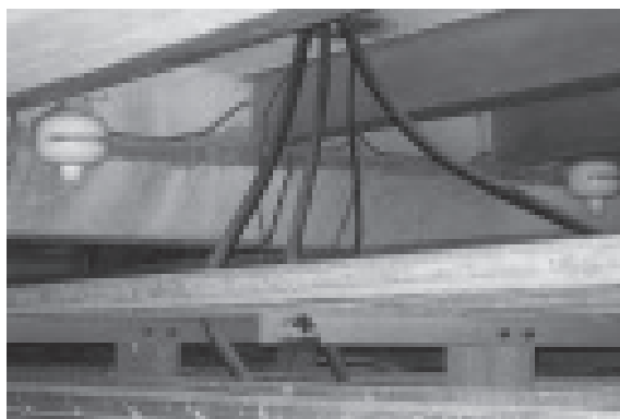
Figure 7 – Substation cables and installed fire/flame detector
