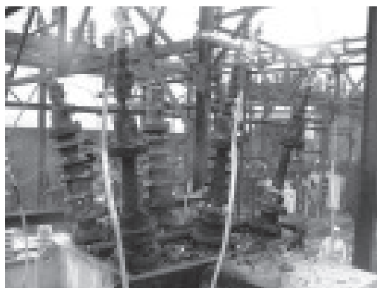
Figure 4 – Failure of 33 kV oil circuit breaker (photo credit: ethw.org)
