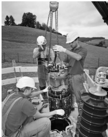
Maintenance of on-load tap-changer
