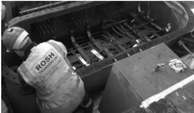
Repair of transformer gaskets
