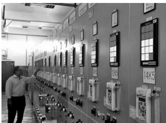
Figure 12 – Typical alarm annunciator in substation
