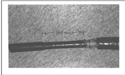
Figure 7: Contraction of MVABC Joint
