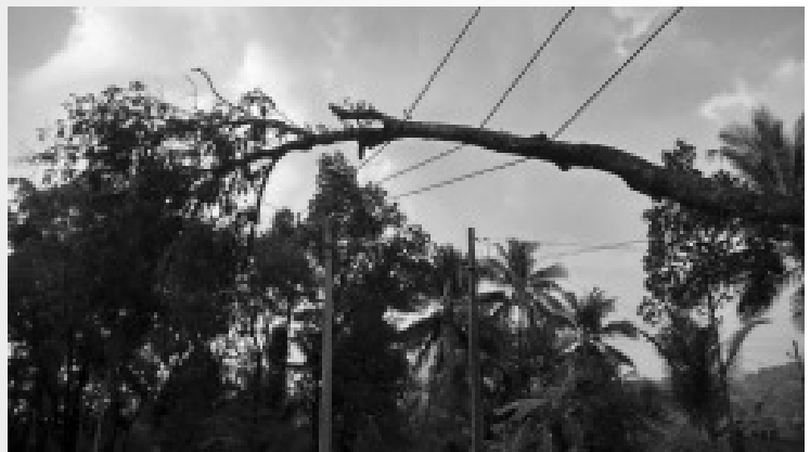
Tree on 33kV Live Line (CC)
