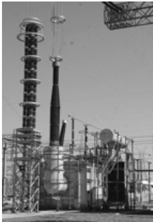
A single-phase 400/1,200-kV auto-transformer at the site
