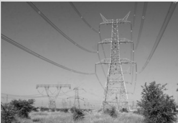
A view of 1,200-kV single-circuit line (left) and 1,200-kV double-circuit line (right).
