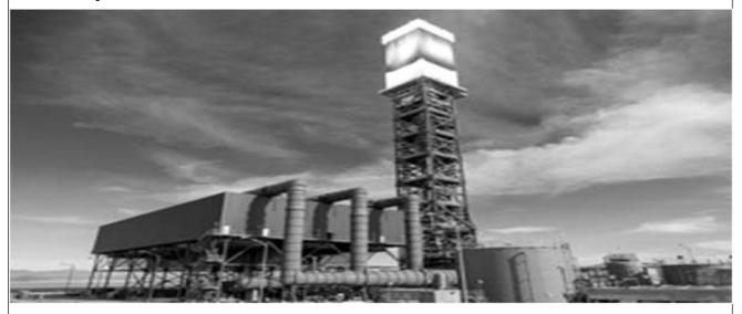
Ivanpah Solar Electric Generating System situated in the Mojave Desert in California is the World's largest solar power plant. An engineering marvel in itself, Ivanpah uses over 3,00,000 mirrors (heliostats) to reflect heat and light from the Sun onto boilers atop three of the towers here. Each of these towers is 150 feet taller than the Statue of Liberty.
