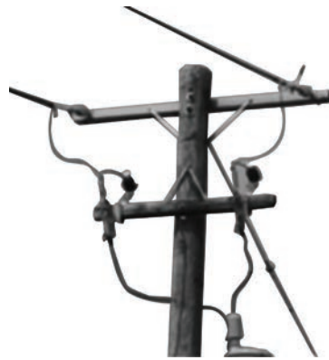
Fig. 4.15 Double-channel Cross-arms
