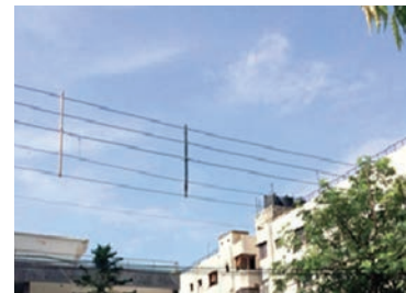
Fig. 4.18 Vertical Line Spacers
