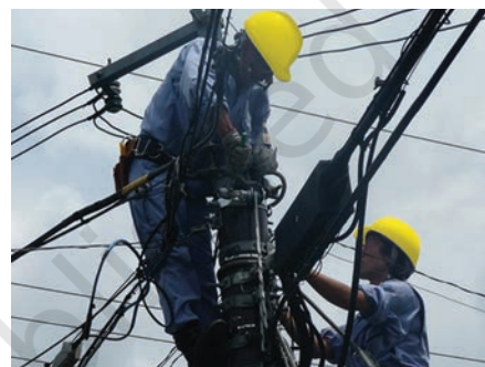
Fig. 4.53 Inspection of Power Distribution Lines
